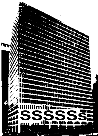
Figure 1. Two Shell Plaza, Houston Texas
