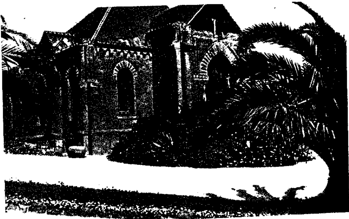
B. Hills of Eternity Cemetery, south of San Francisco. All firm gables thrown out. Parapets thrown in on roof. A. C. L.
