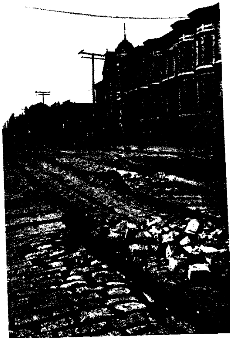
B. Looking south on Howard Street from near Seventeenth Street. Compression flexure of car rails. G. K. G.
