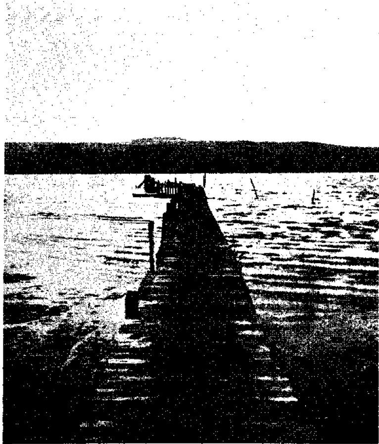
A. Martinelli's pier at Inverness. Originally straight; shifted and broken by earthquake. Repaired before photograph was taken. G. K. & G.
