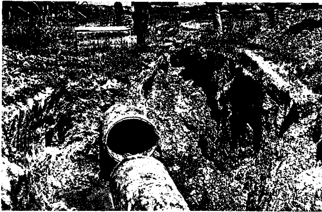
A. Rupture of 30-inch water-pipe by fault. Northwest of San Andreas Lake, A. O. L.
