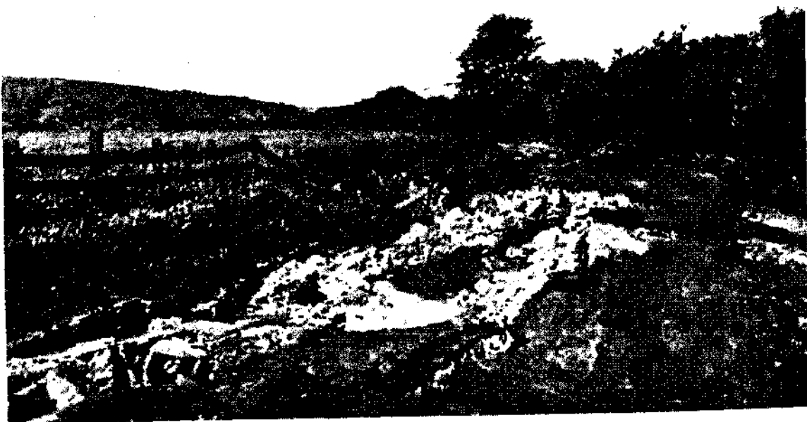
B. Destruction of road due to subsidence of ground toward Salinas River. H. K. Brown. A. C. L.
