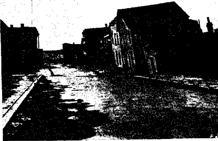
A. Looking along Dore Street from Brannan toward Bryant, Larger undulations near Brannan, Dore Street is on site of an arm of Mission Creek. H. O. W.
