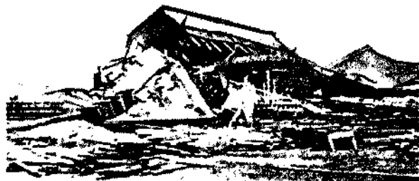
E. Haywards. Wreck of buildings by earthquake of 1868.
