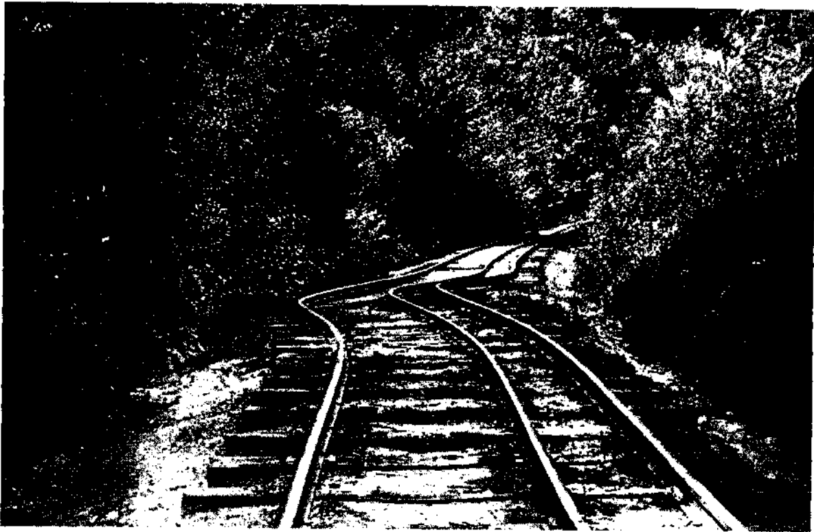
A. Shortening of railroad track between Los Gatos and Santa Cruz. Oh Ai Wi
