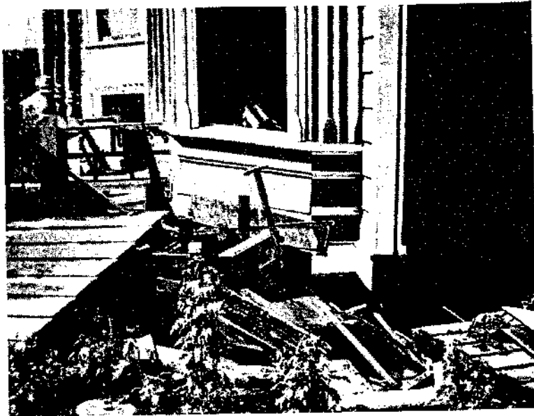
A. House moved 7 feet by collapse of underpinning, Santa Eosa. E. S. H.
