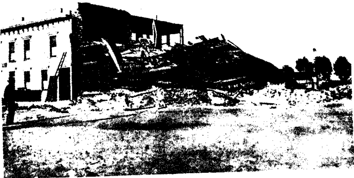
B. Wreck of 2-story brick buildbg, San Mateo. Per J. C. B.
