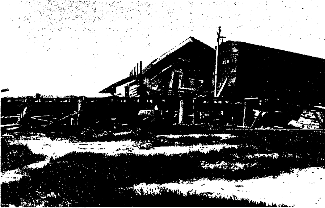
A. Moss Landing. Inching of ground toward Salinas Eiver, to left, carried piles from "beneath bridge timbers and caused bridge to collapse. Displacement 9 feet. A. G. L.
