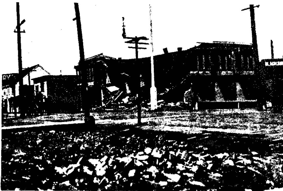
B. Wreoked buildingSi Fort Bragg. Looking northwest!
