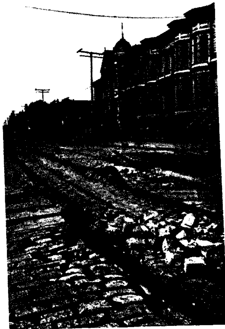
B. Looking south on Howard Street from near Seventeenth Street. Compression and flexure of car rails. G. K. G.
