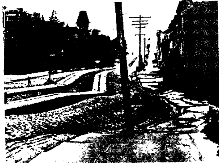
B. Slip of a fill on Union Street, just west of Steiner Street, San Francisco. H. O. W.
