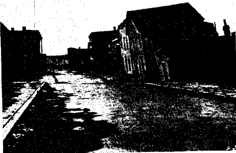
A. Looking along Dore Street from Brannan toward Bryant, Larger undulations near Brannan, Dore Street is on site of an arm of Mission Creek. H. O. W.
