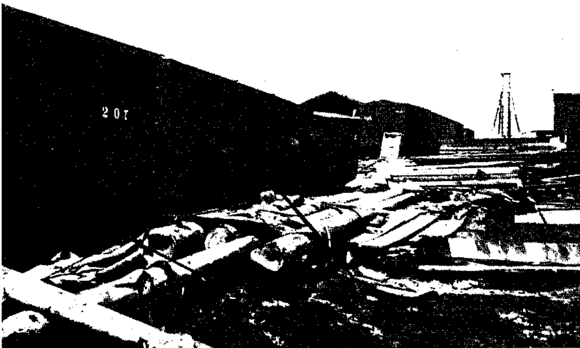
B. Moss Landing. Deformation of surface due to Inching of ground toward Salinas Ei?er. A. O. L.
