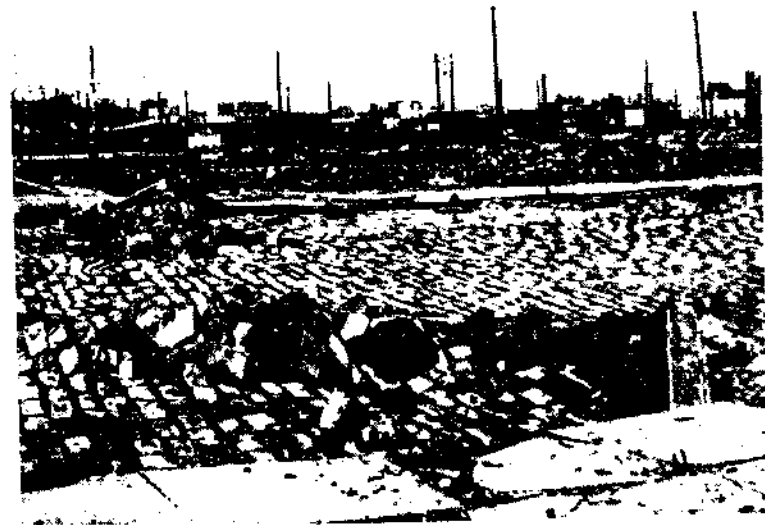
D. Moss Street, between Folsom and Howard Streets, San Francisco. Paving blocks arched by compression along sinuous crest, curbing thrown into an inverted V. H. O. W.
