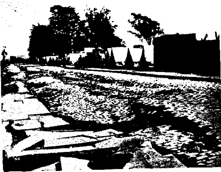
A. Columbia Street, just south of Folsom Street, San Francisco. Slumping, depression, and farrowing of block pavement. H. O. W.
