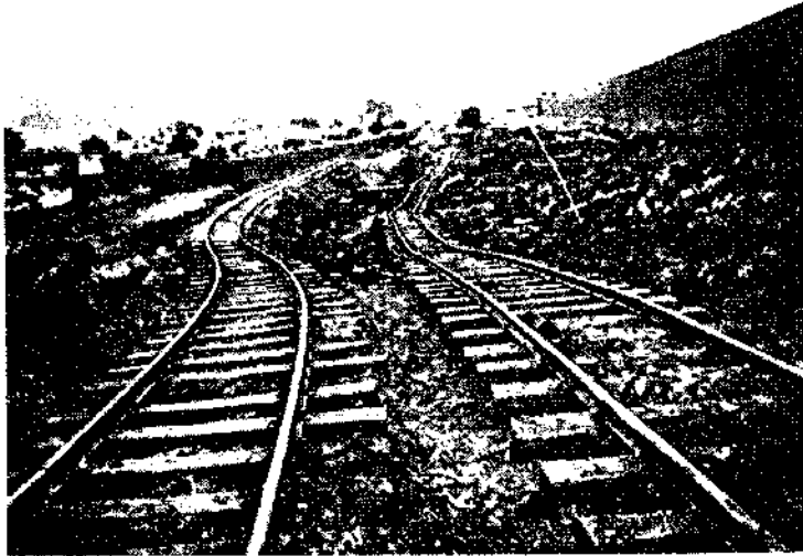
A. Earth-slip north of Tomales, carrying railway roadbed with it. Track was straight before earthquake. R. S. H.
