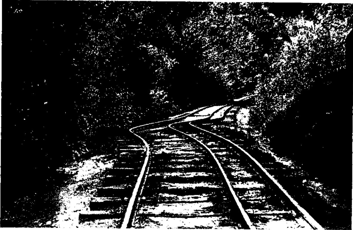
A. Shortening of railroad track between Los Gatos and Santa Cruz. Oh Ai Wi
