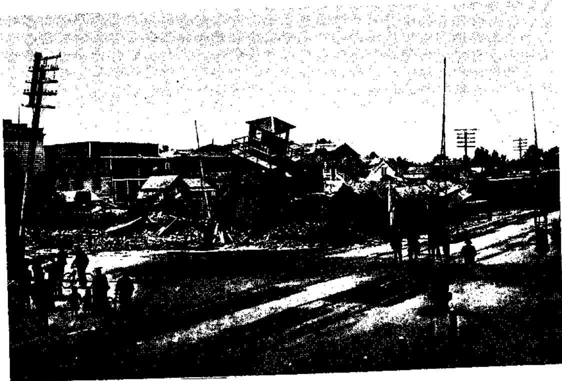
A. Wreck of 1-story brick railway warehouse, Beaufort, N. C. Per J. O. B.
