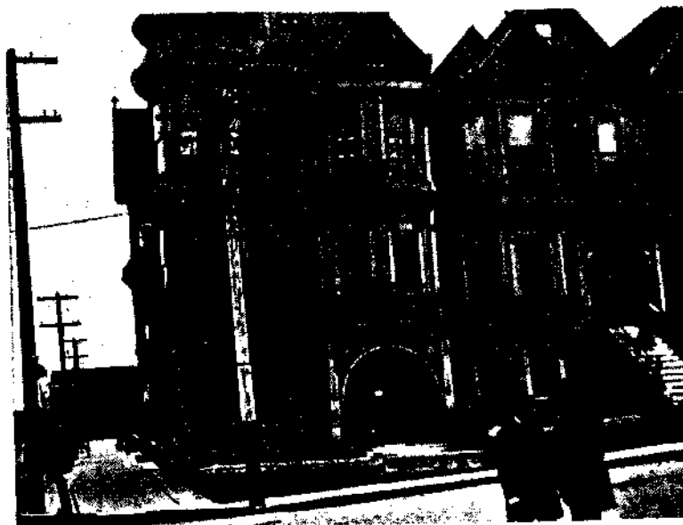
D. Southwest corner Portola and Waller Streets. Buildings have shifted down hill slightly, upper parts more than lower. H. O. W.
