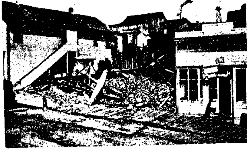
A. Point Arena. Brick house destroyed j wooden houses little affected. P. E. H.
