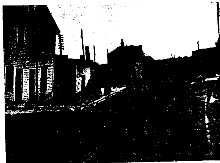
B. Dore Street, near Brannan, Vertical difference between crest and trough of undulations, 5 feet. H. O. W.
