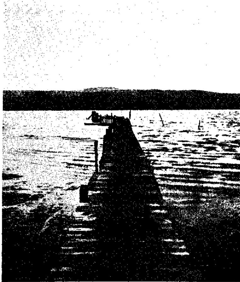
A. Martinelli's pier at Inverness. Originally straight; shifted and broken by earthquake. Repaired before photograph was taken. G. K. & G.
