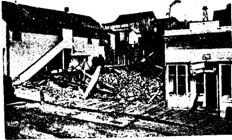
A. Point Arena. Brick house destroyed j wooden houses little affected. P. E. H.
