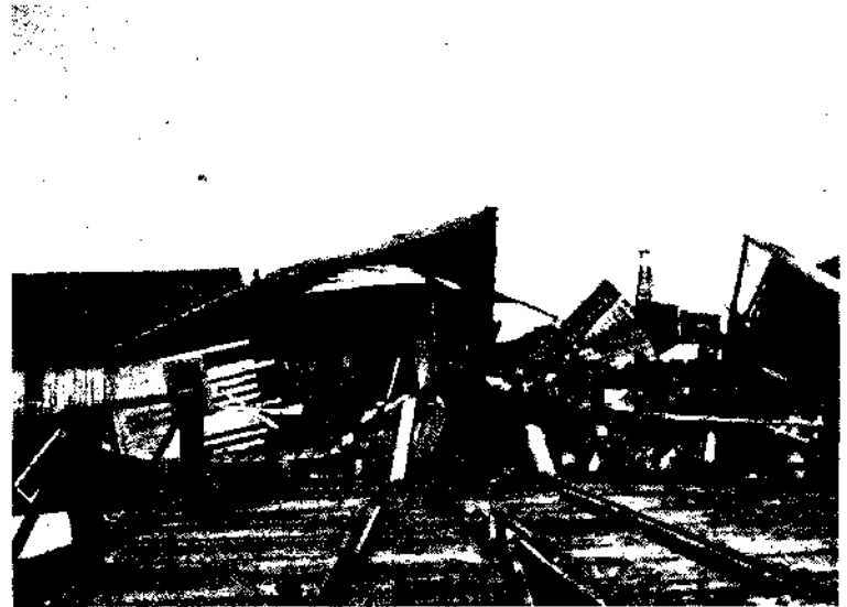
D. Hoss Landing. Wreck of wooden warehouse. G. B. B.
