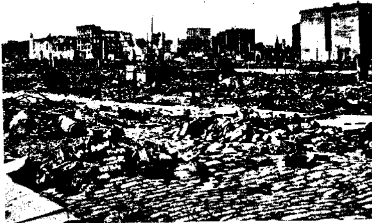
C. Buss Street, between Polk and Howard Streets, San Francisco. Paving blocks forced up into sharp arches and dislodged by compression. H. O. W.
