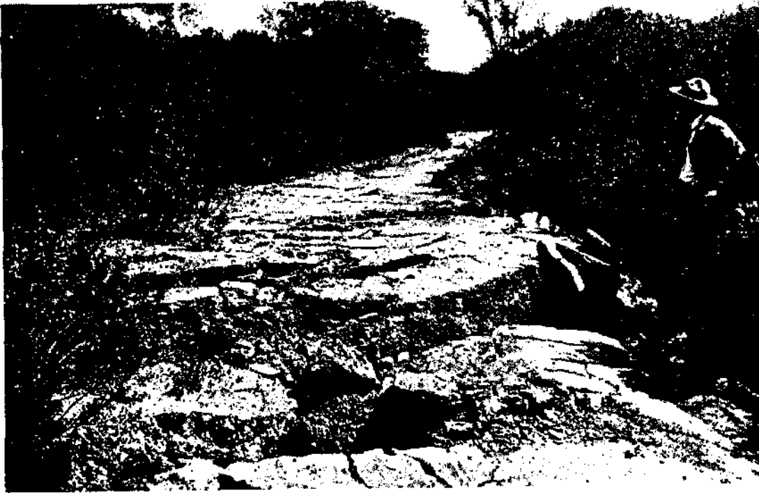
A. Offset of Alpine road 5 miles west of Staaford University. Per J. O. B.
