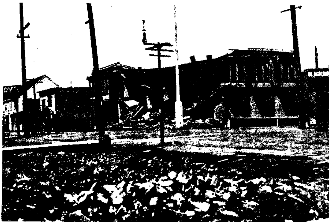
B. Wreoked buildingSi Fort Bragg. Looking northwest!
